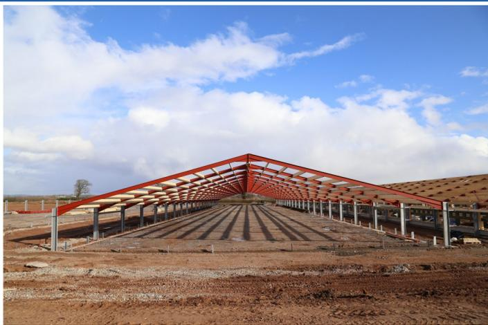
Due to the geographical location of the site and the ground conditions 18,000 square metres of ground was stabilised with a 30% CBR replacement layer of lime. This resulted in an 85% reduction in HGV deliveries that would otherwise have been required to bring in stone to the site.
