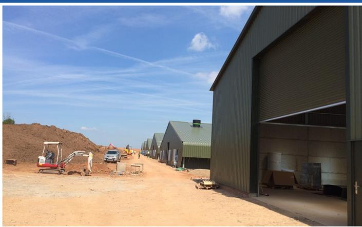
Formation of the 8,746 square metre external concrete aprons and access road along with the 19,542 square metres of internal flooring was carried out by Knights Concrete Flooring Division. The external areas were given a brush finish with the shed internal floors being power floated smooth to allow for easy wash out. 1,641 metres of concrete mass-filled walls were also formed in the control room areas of the units.
