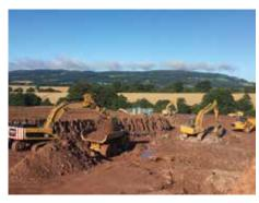
rain eased, our excavators got to work. Early into the excavations, our teams hit a large amount of rock. Provision was quickly put into place to utilise this existing rock and a crusher was brought onto site. The rock was then able to be recycled in the makeup of the site formation and will further be utilised on future projects.
