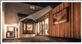
THEN & NOW Main image: Work gets underway Inset: The new entrance
