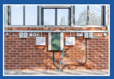
Traditional brickwork and blockwork followed to allow the installation of the glazing and the integrated GRP guttering to the centre of the greenhouse. All the glazing was finished with lead flashings, in keeping with the style and aesthetics of the build.
